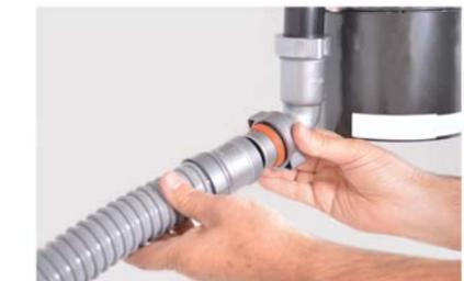
Connect the hose to disposal elbow. You may need to place the remaining sink elbow (c) between the hose and disposal elbow.
