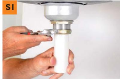
If you have an existing tailpiece in place, remove it by untightening the locking nut with adjustable pliers.
