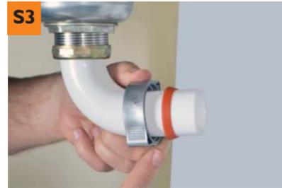
Slide slip nut (g) and orange washer (e) into the tailpiece elbow, with the conical side of washer facing out. If you need to connect a dishwasher drain hose, continue to step S4. Otherwise, go to step S5.
