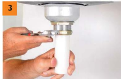
Untighten the strainer locking nut, you may need adjustable pliers. Remove existing tailpiece.
