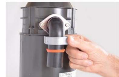
Slide slip nut and orange washer into elbow, with the conical side of washer facing down.
