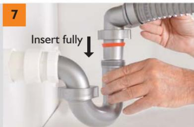
Insert hose section (a) into P-Trap, with conical side of washer facing down. Make sure the hose section goes in all the way. Tighten slip nut **loosely**, allowing the section to swivel to fit in space.
