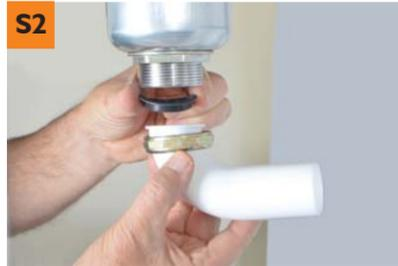
Place the tailpiece washer (f) in the top of the tailpiece elbow (i) and slide into strainer locknut. Insert the tailpiece elbow into the strainer and tighten locknut loosely, allowing elbow to swivel. This will allow the hose to accommodate properly.
