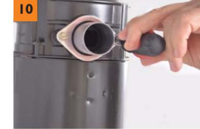
Insert tailpiece (h) into disposal outlet, followed by the metal flange of your disposal (some disposal models may have a clamp or other accessory). Tighten flange screws with screwdriver.
