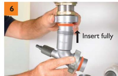
Insert the regular elbow, or elbow with dishwasher drain branch (c) if you need to connect a drain hose to the Snappy Trap. You may also use the elbow with dishwasher drain branch as a regular elbow by leaving the black cap on at all times.
