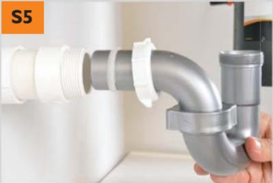
Remove the existing slip nut and washer from the marvel adapter in the pipe entering the wall and slide them on the P-Trap, with the conical side of the washer facing out. Insert P-Trap into the marvel adapter and tighten slip nut firmly. We have included an extra slipnut washer (e).
