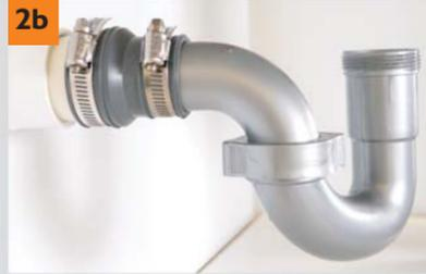
If you don't have a marvel adapter in place, use the wall coupling (d) included. (The larger side of the coupling connects to wall drains with approximately a 2" exterior diameter). Insert P-Trap through coupling and into the pipe, adjust metal clamps firmly.
