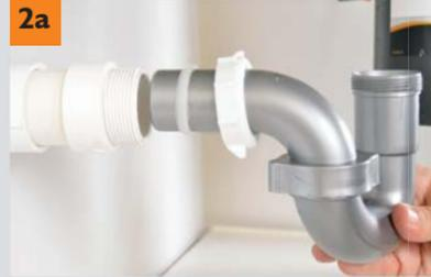
Remove the existing slip nut and washer from the marvel adapter in the pipe entering the wall and slide them on the P-Trap, with the conical side of the washer facing out. Insert P-Trap into the marvel adapter and tighten slip nut firmly. We have included an extra slipnut washer (e).
