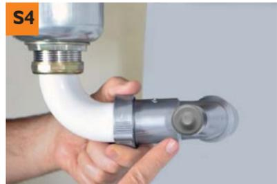
To connect a dishwasher drain hose, insert the elbow with dishwasher drain branch (c) into the tailpiece elbow, place it horizontally. Then, proceed to S5.
